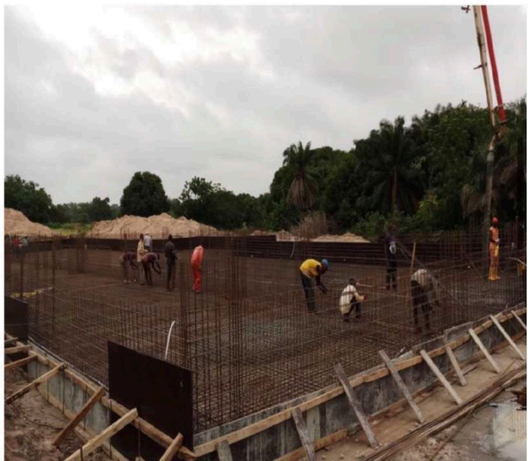
*Nigeria/Kontagora Dormitory Building 3000m2
