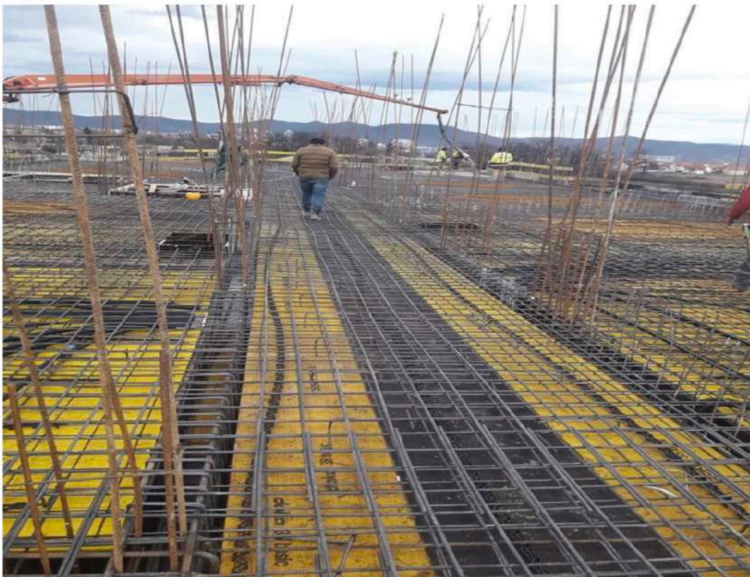
Kraljevo-4000m2-Rough Works Project-As Finised
