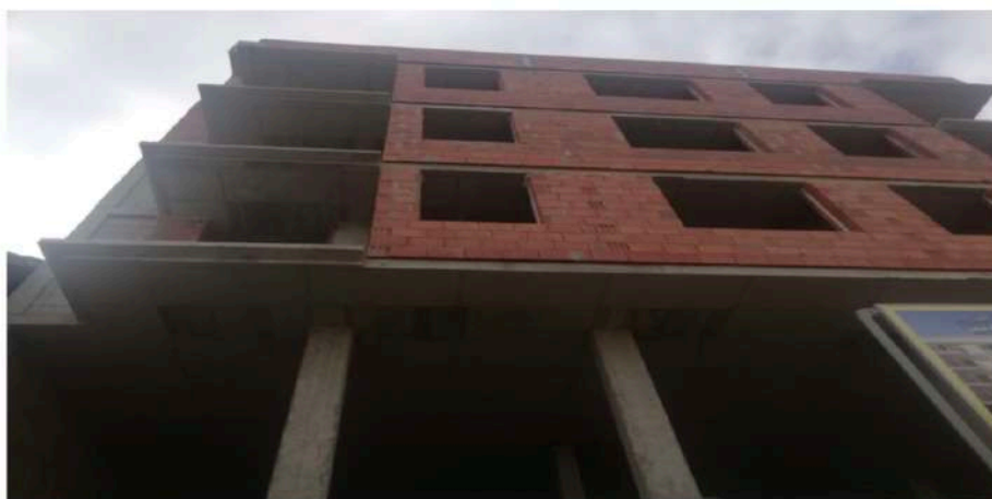
NoviSad-2000m2-Roughly Works Project-Finished
