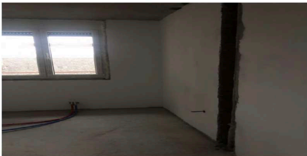
Novisad-10.000m2-Finishing Works Project- Finised
